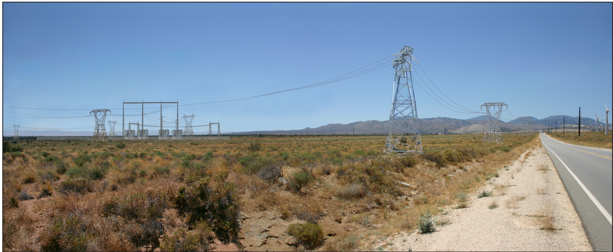
B Substation One as seen from KVA Seg 3-2.
